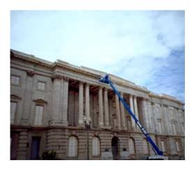
Low-to-medium-pressure steam (hot-pressurized water washing) is a gentle method of softening heavy soiling deposits and cleaning historic marble. Photo: NPS files.
