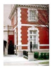
The decorative trim on this brick builing is architectural terra-cotta intended to simulate the limestone foundation. Photo: NPS files.
