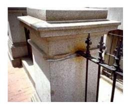
The iron stain on this granite post may be removed by applying a commercial rust-removal product in a poultice. Photo: NPS files
