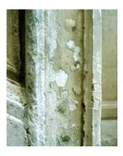
This clear coating has failed and is pulling off pieces of the stone as it peels. Photo: NPS files
